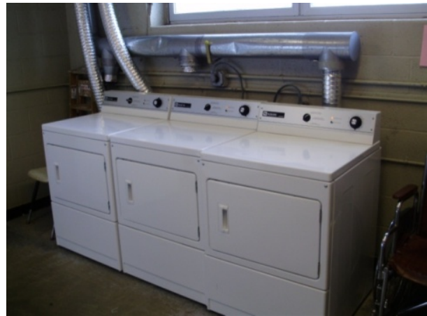
Three new washers in Haven Center
